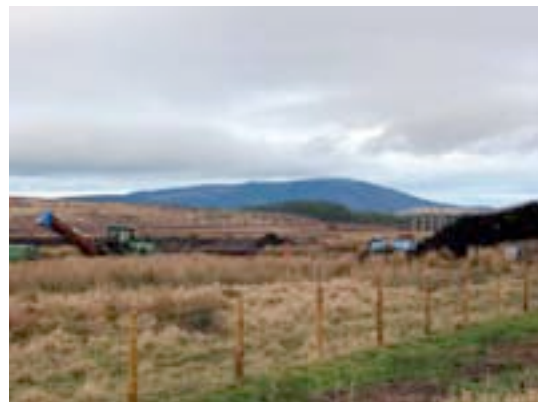
Machinery and stockpiles of excavated peat
